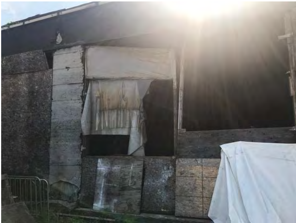
Figure 2: Workshop structure on site.
