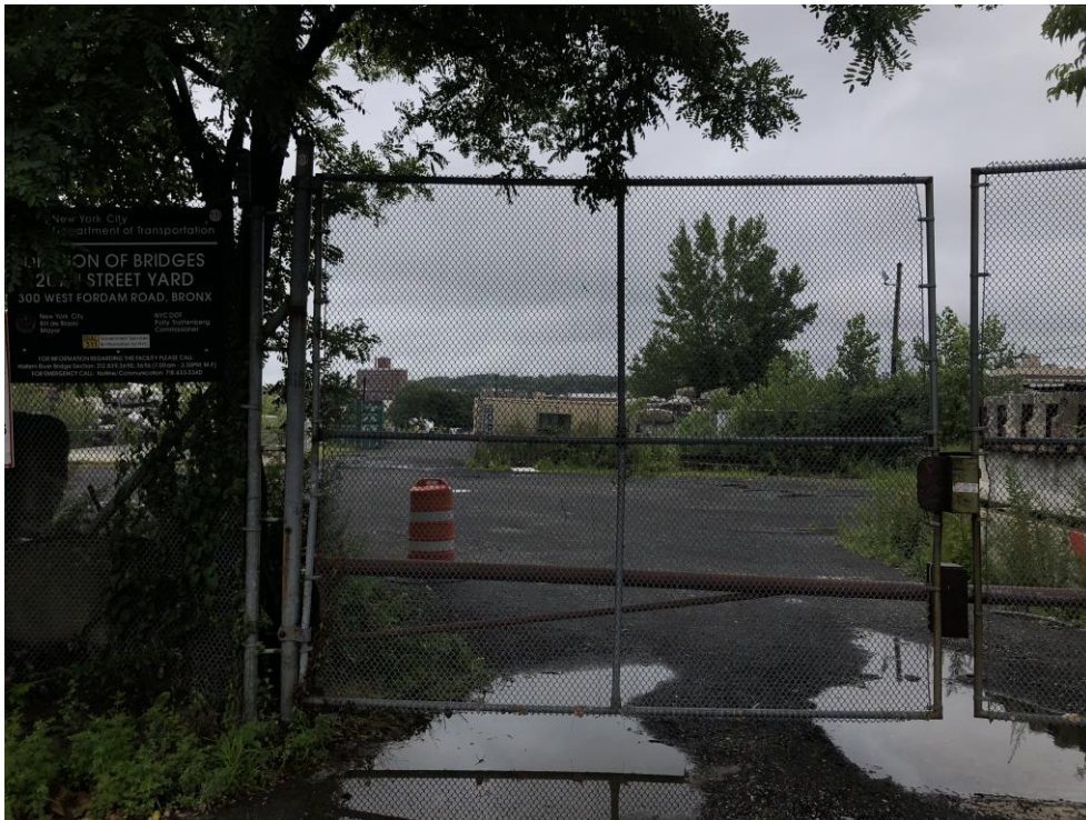
Photograph 16: View of adjacent NYCDOT – Division of Bridges 207 th Street Yard, southwest of Subject Property; facing west.
