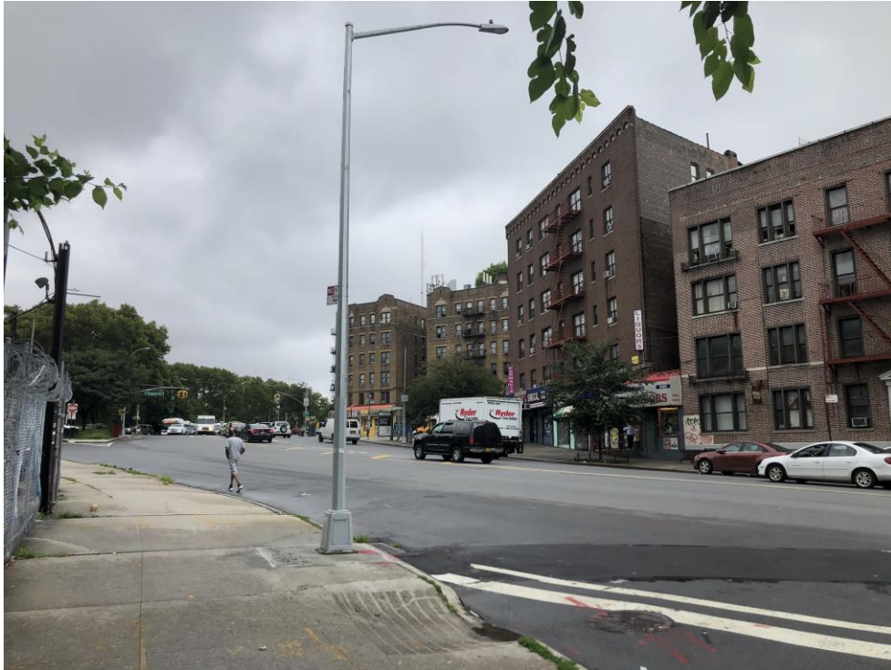
Photograph 17: View of adjacent and up-gradient residential and commercial properties east of the Subject Property, across the Major Deegan Expressway; facing northeast.
