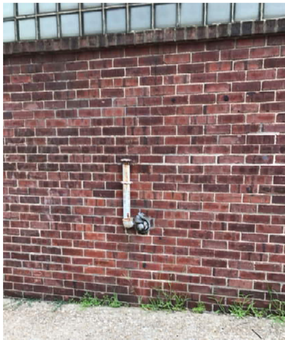
Photo 12: View of the fill port and vent pipe on the southern side of the Subject Property building, facing north
