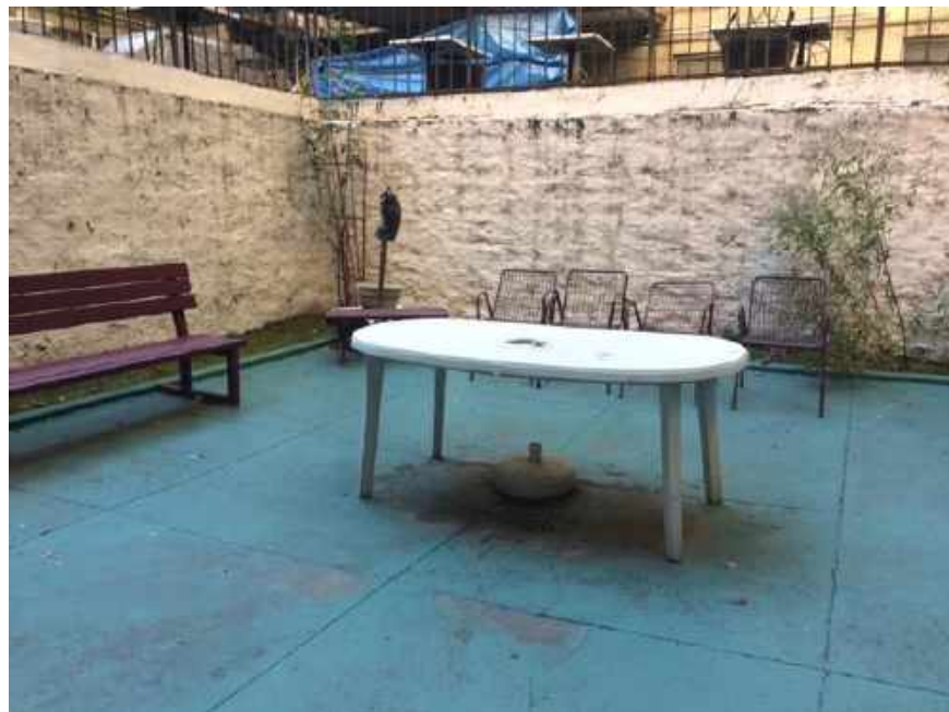
Photograph 16: View of the exterior patio located behind the Lot 60 building, facing south.
