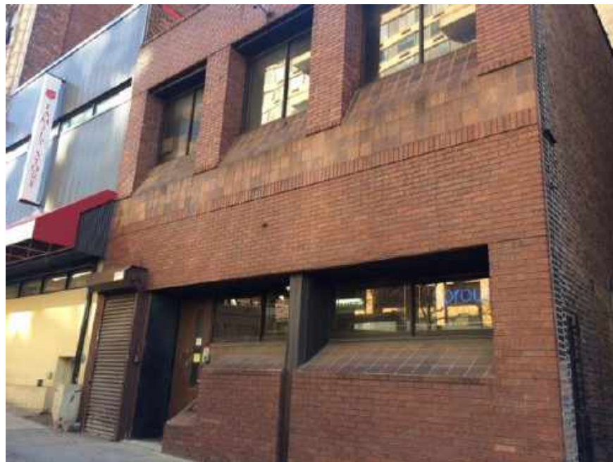
Photograph 10: View of the building located on Block 1243, Lot 60, facing southeast.
