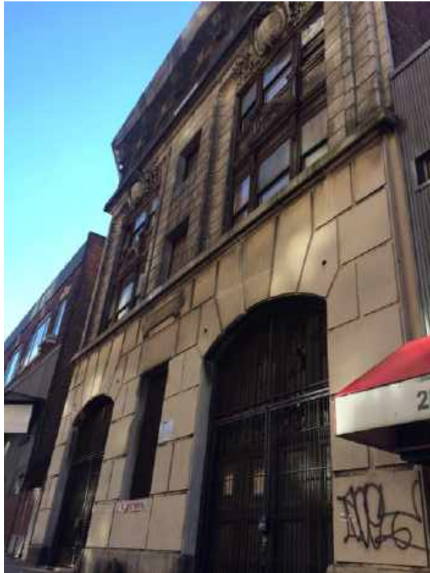
Photograph 1: View of Block 1243, Lot 57, facing southwest.
