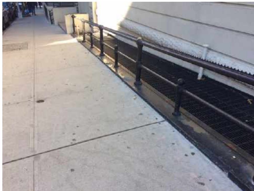
Photograph 20: View of vent and fill port located in front of a southern adjoining property, facing south.
