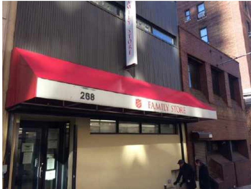
Photograph 5: View of the Block 1243, Lot 59 building, facing southeast.
